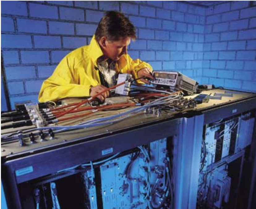
The R&S®NRT during installation of a mobile radio base station
